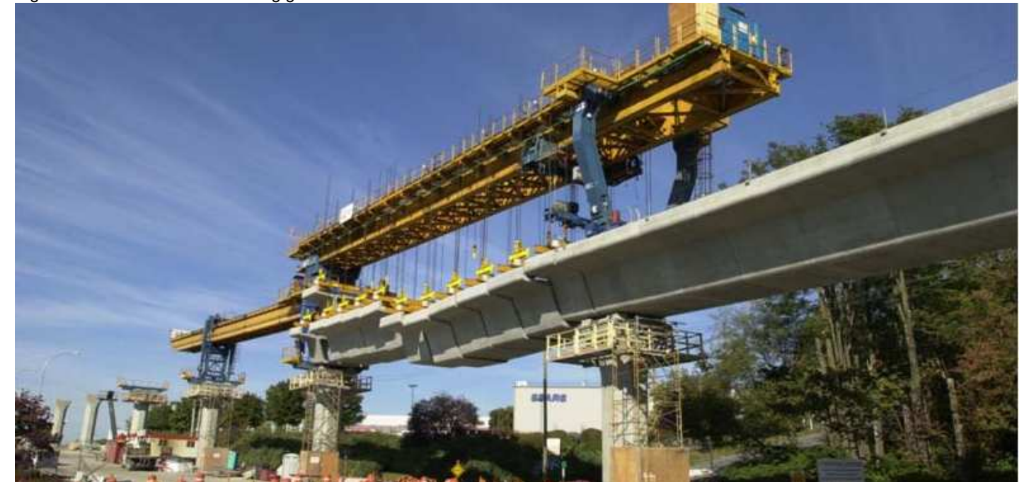
Figure 17: Overhead self-launching girder
